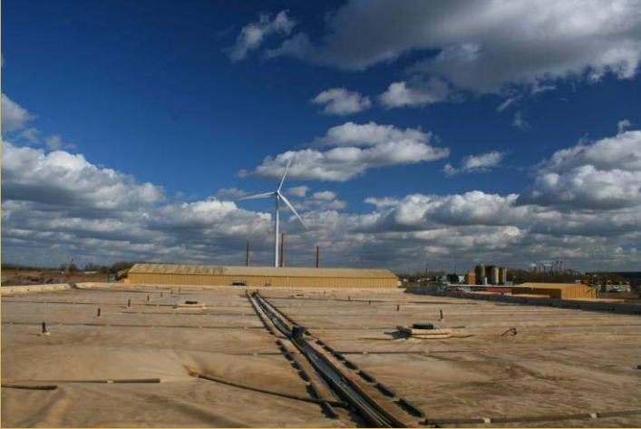
Installed Cover showing central float and ballast arrangement
