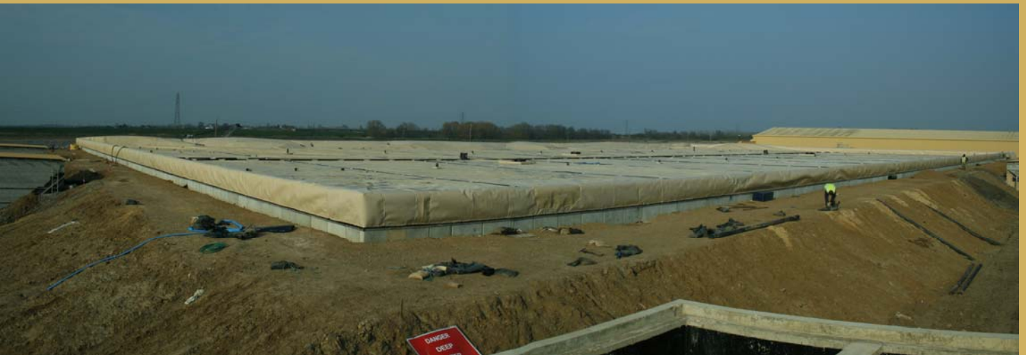
Completed Geomembrane Cover
