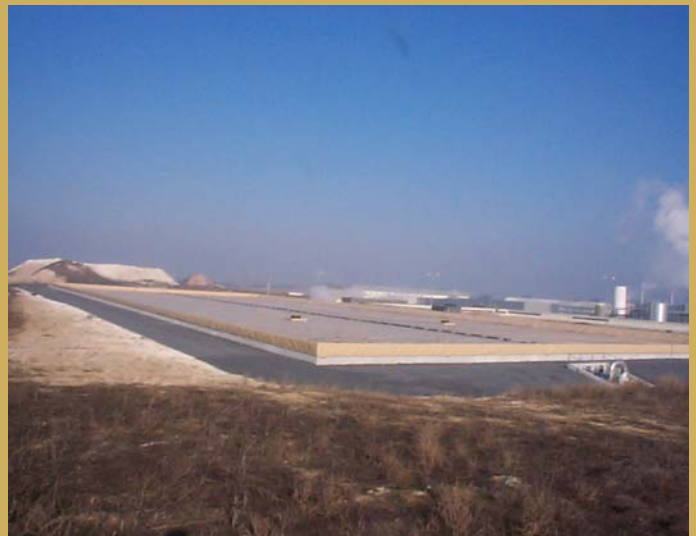
Geomembrane Cover Complete
