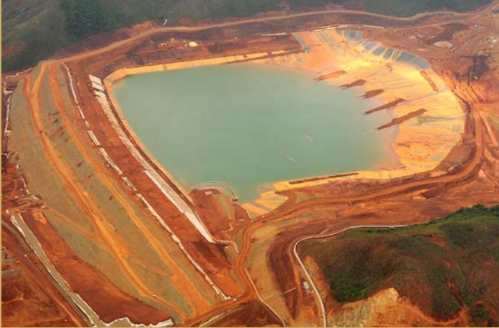
Tailings Management Facility
