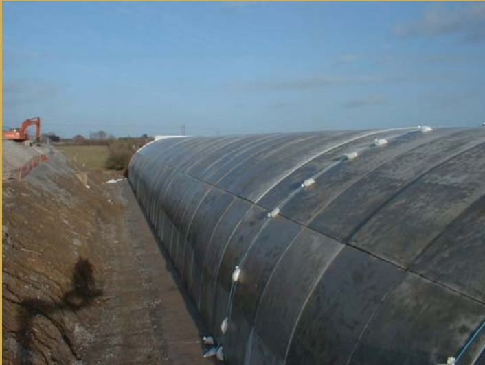
Matiere Pre-cast Arch Installed
