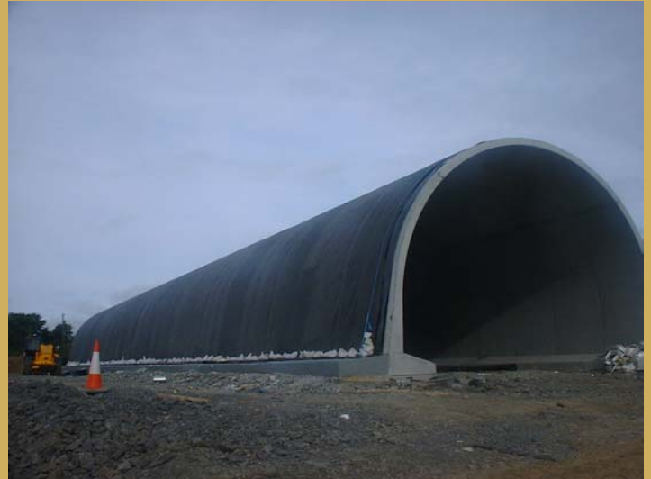
Waterproofing HDPE liner Installed
