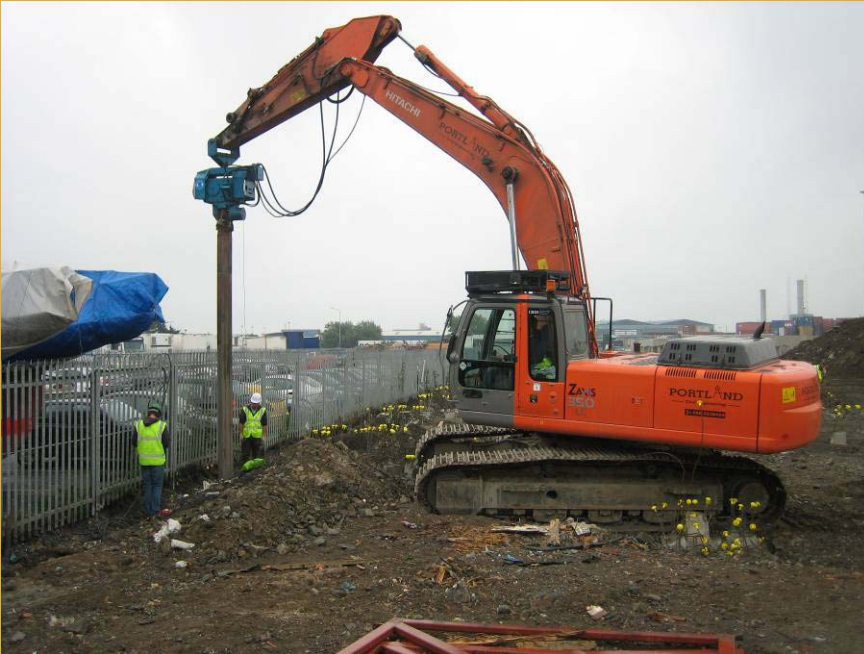
Driving Gas Vent Chimneys
